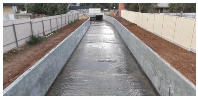
Channel construction through to completion
